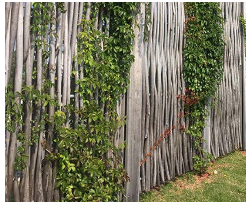
Acoustic willow wall works provides absorption and sound insulation
