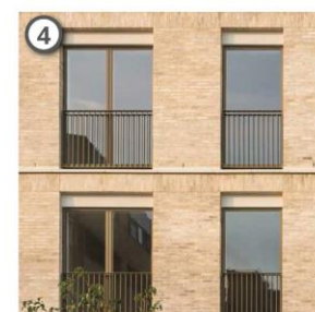
Window brick header
