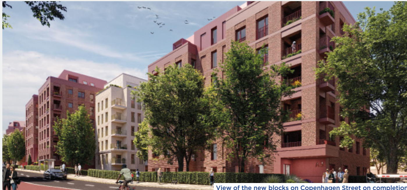
View of the new blocks on Copenhagen Street on completion
