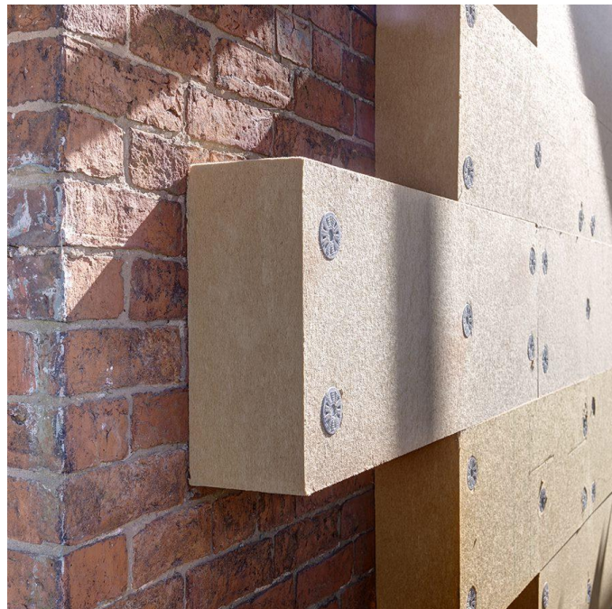
External wall insulation in deck access to improve thermal efficiency and aspect
