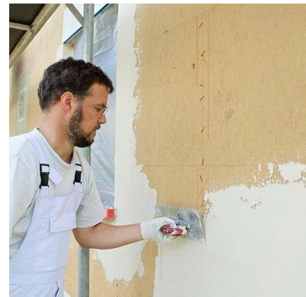
External wall insulation in deck access to improve thermal efficiency and aspect
