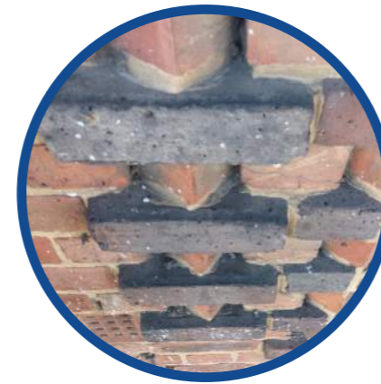
Existing brick details
