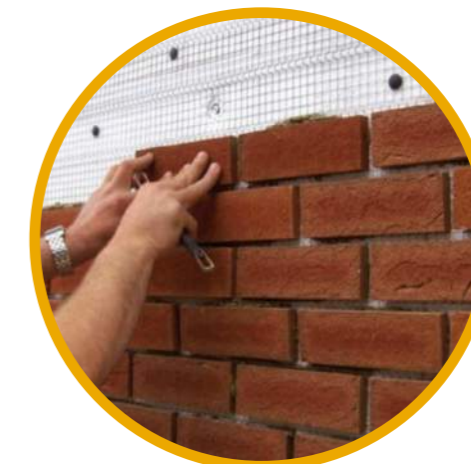
3 - Brick slips are applied
