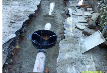
Front of Blackmore House drainage run install
