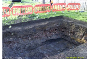
Carnegie Park ground drainage initial inspection
